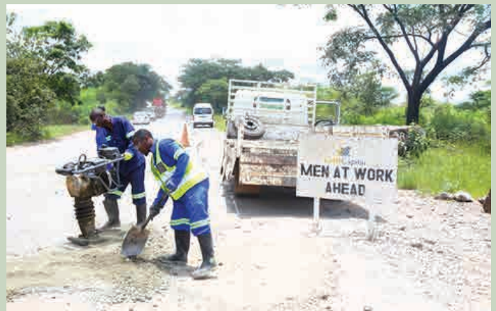
Lubambe employees patching potholes on the international road in Chililabombwe leading to Kasumbalesa Border Post
