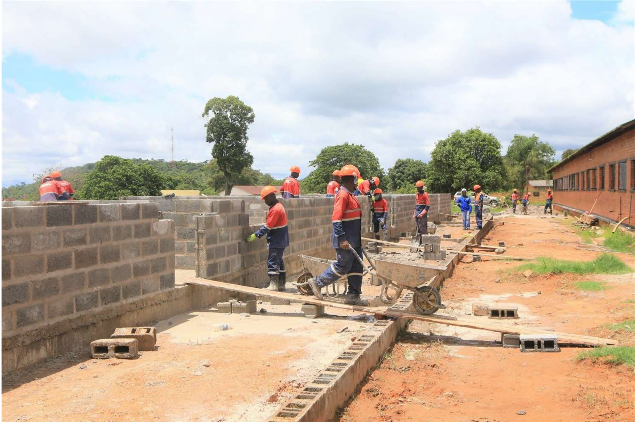
Construction of the 1 by 4 classroom block
