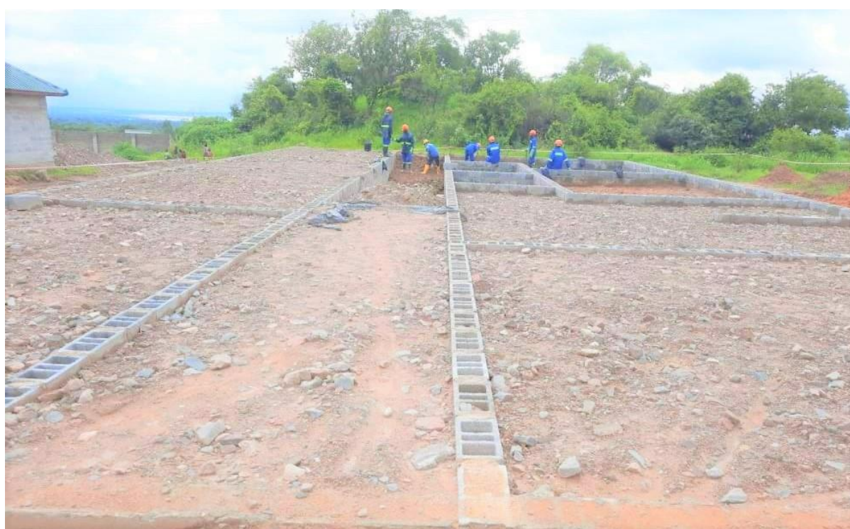
Construction of maternity wing at foundation level
