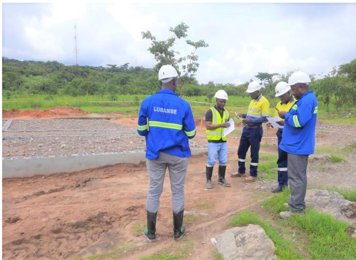
The Lubambe team at the construction site
